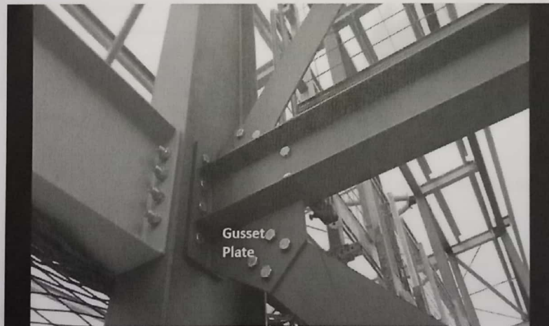
(c) Bolted connection with gusset plate
