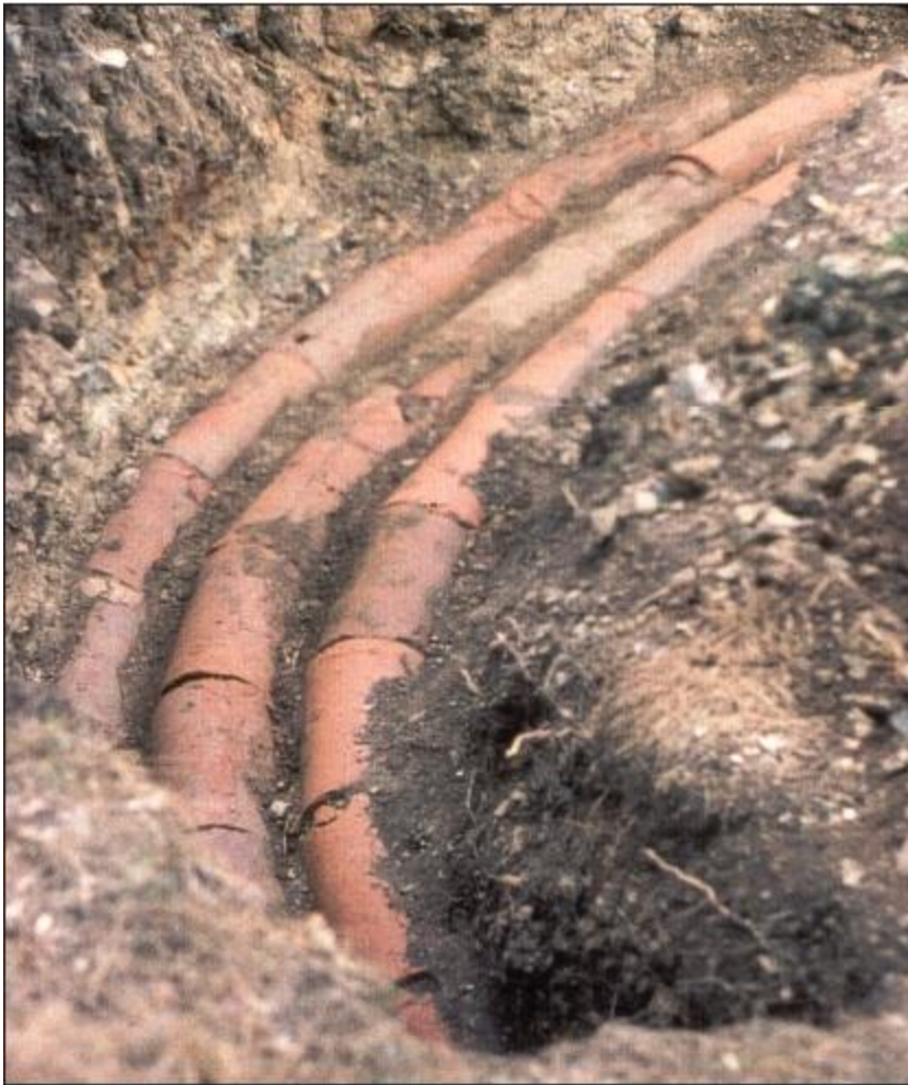
Segment of Pergamon pipeline. Each clay pipe section was 13 to 18 cm in diameter.
