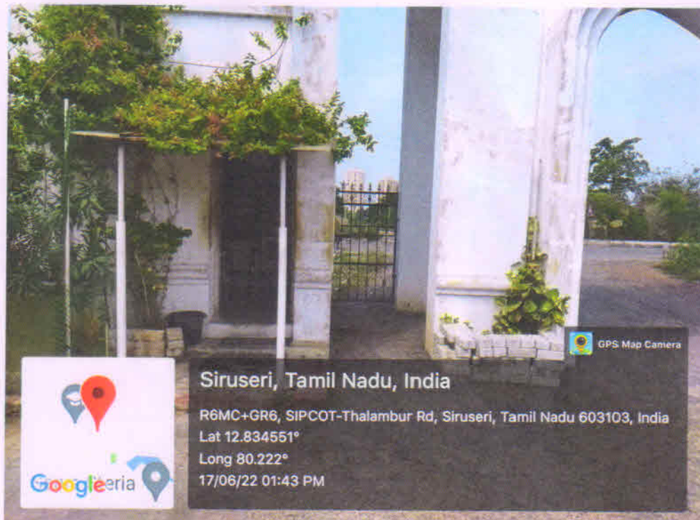
Security Room at the campus entrance
