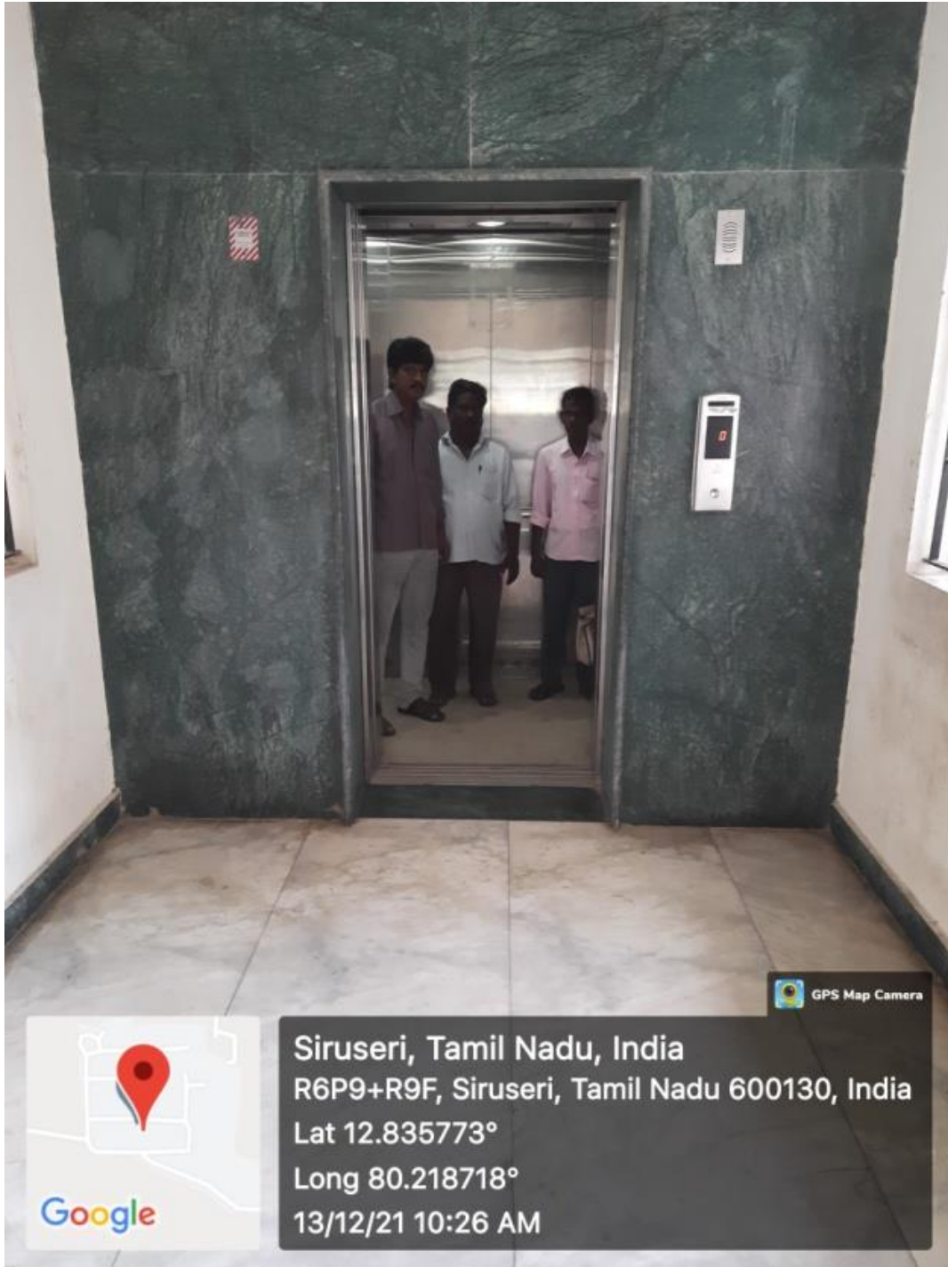
Lift at Main Building Ground Floor
